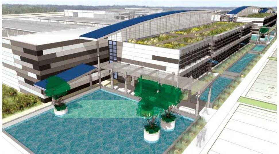
*Water harvested from the roof is treated and stored in open "pool" features outside the building for use in the evaporative cooling system.*
